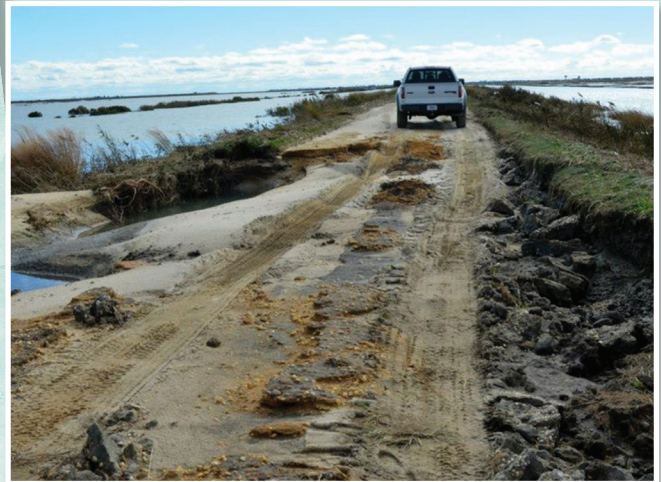
Example of erosion along south dike of Wildlife Drive. Photo: Edwin B. Forsythe National Wildlife Refuge Facebook homepage.
